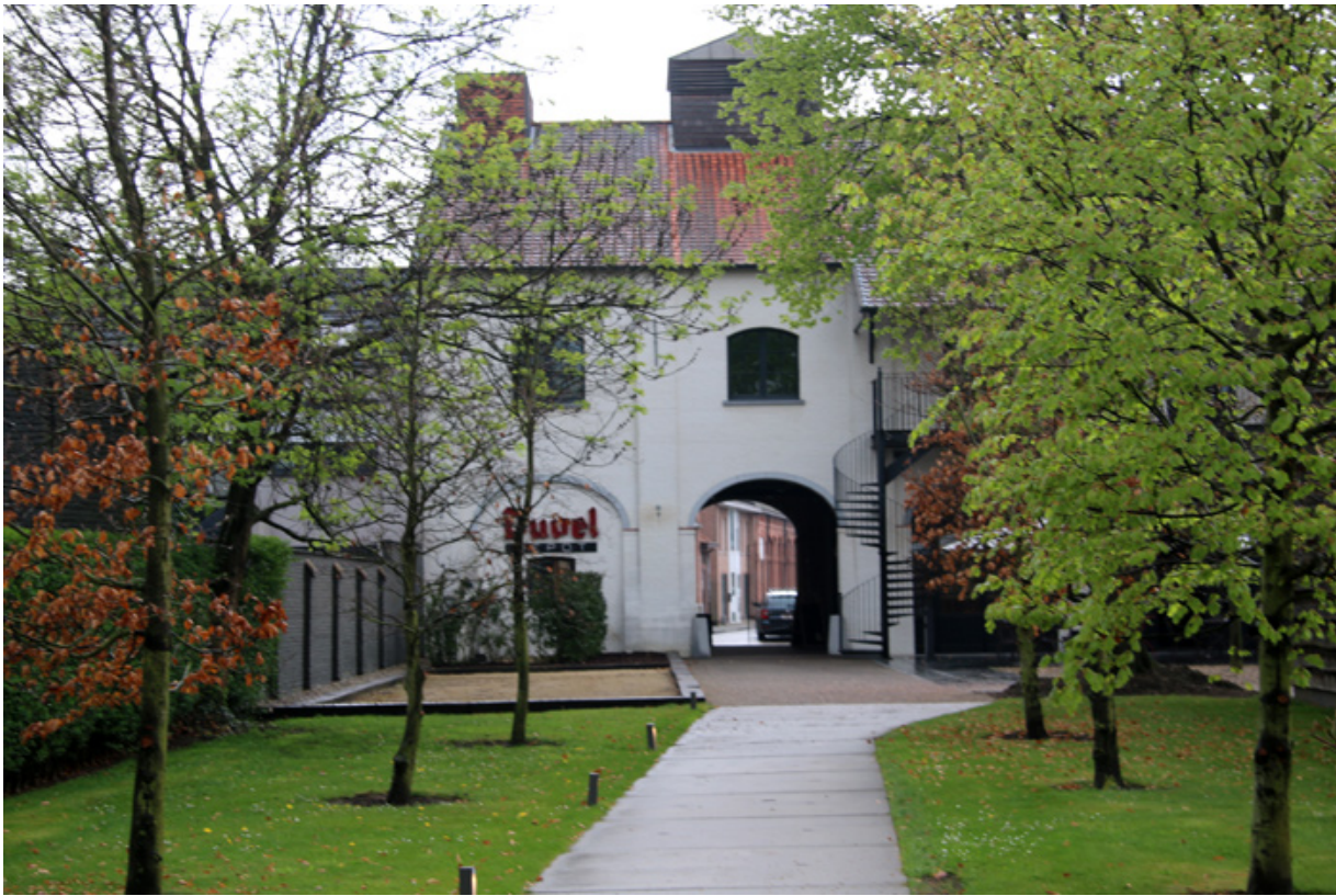
Duvel hospitality building
